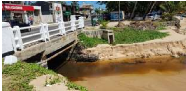
Figure 11: Mawakada canal is connected to the sea by cutting the sandbank
